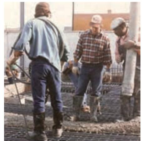
**Figures 19 and 20.** The reinforcement rod grid supports the concrete vault walls, floor and ceiling. At right, the crew begins the concrete pour.
