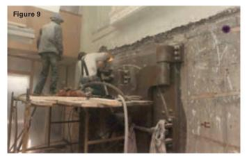
**Figures 7-9.** It took the crew seven days of taking turns with the jack-hammer and the torch to cut through the wall. This was done through a cloud of thick dust and smoke. It was hard to breathe or see, even though fans were running all day to move the air outside.
