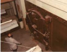
**Figures 4 and 5.** The door, which, again, was covered in rust, faced the bank's lobby. The job was to remove the door from the building in Chicago; take it to the shop in St. Louis for restoration; and re-install it in a new bank.
