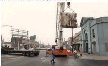
Figure 18. The crane had to lift the vault door about 30 feet in order to clear the telephone lines.
