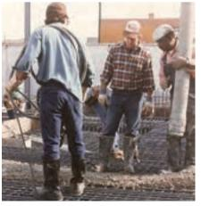
**Figures 19 and 20.** The reinforcement rod grid supports the concrete vault walls, floor and ceiling. At right, the crew begins the concrete pour.
