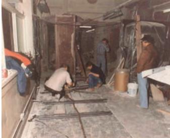
Figures 11 and 12. We kept 1-inch-diameter rollers in close groups of three about three feet apart. Except for the occasional binding, the hallway stretch went well.
