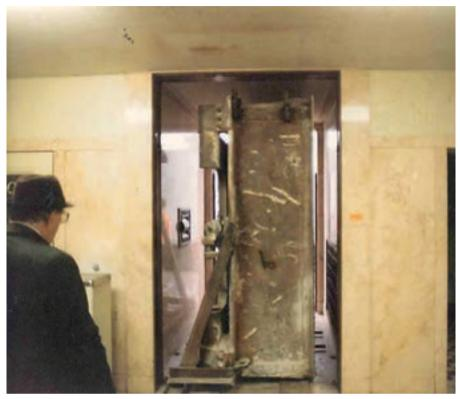
**Figure 13.** When the door was originally measured for height, it was before the frame had been fully exposed. Upon re-measurement, the center was noticeably taller.
